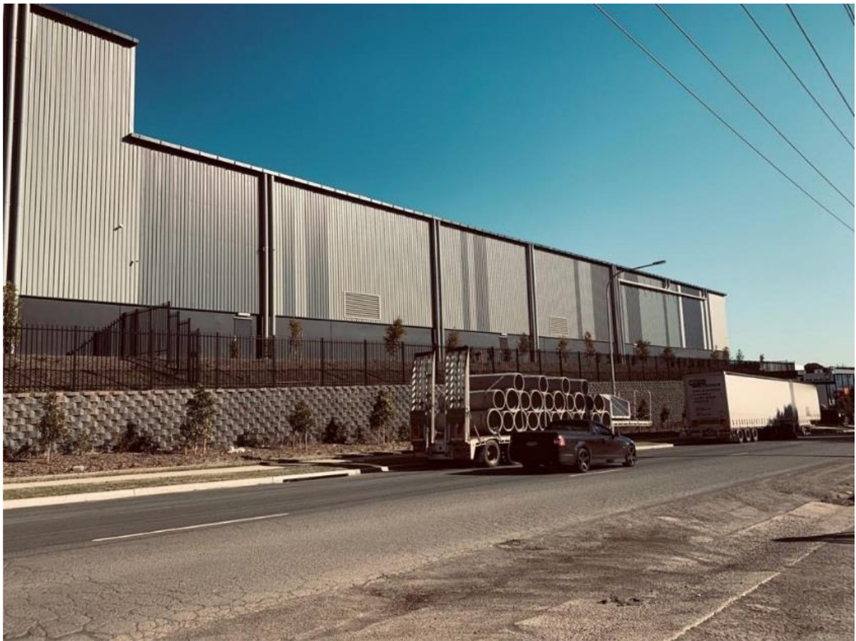
Figure 3 & 4 – 5-35 Yarrunga St – solid reinforced elevated retaining wall on boundary.
